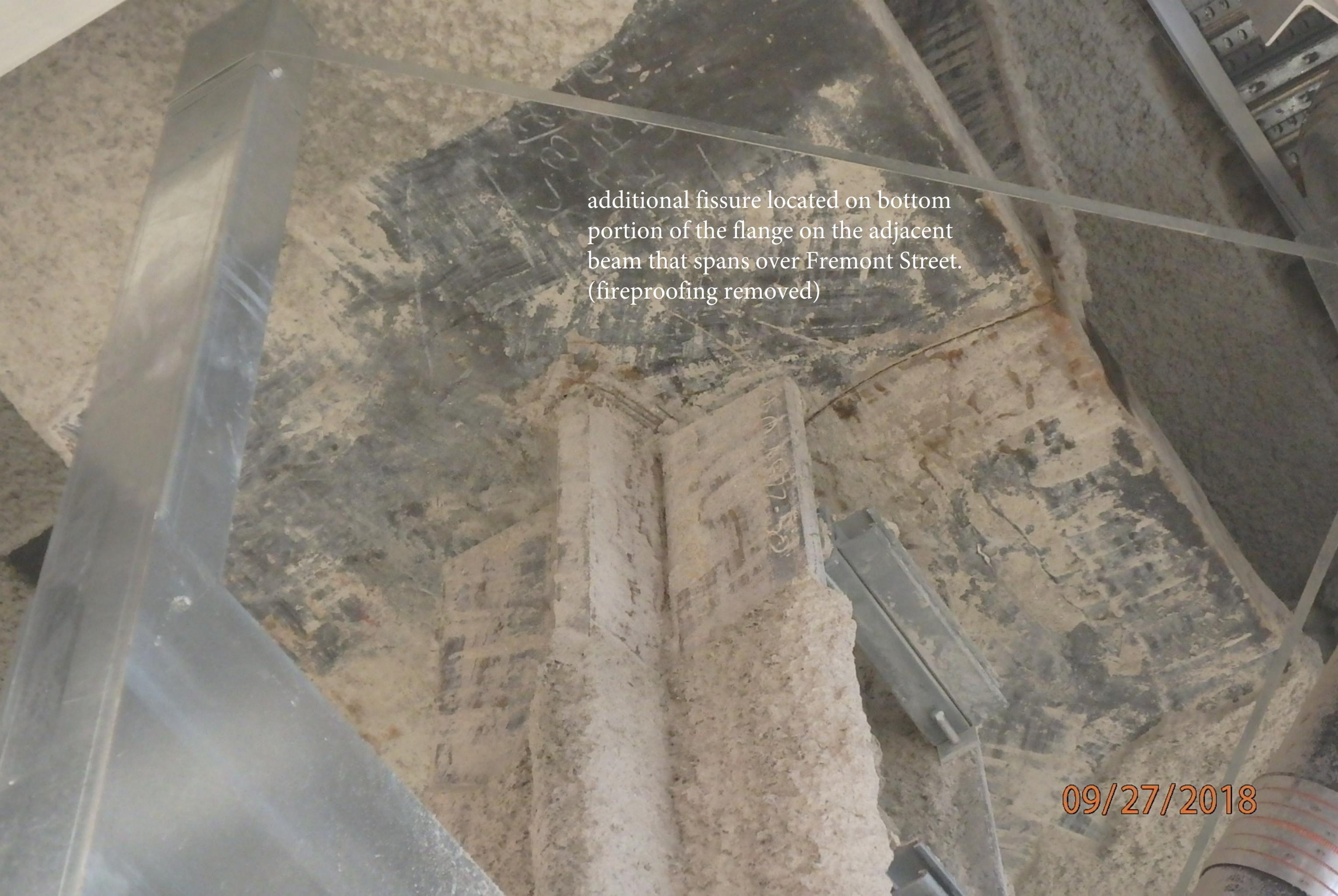
additional fissure located on bottom portion of the flange on the adjacent beam that spans over Fremont Street. (fireproofing removed)
