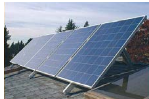
Example of roof mounted photovoltaics panels which generate electricity from the sun's energy.
