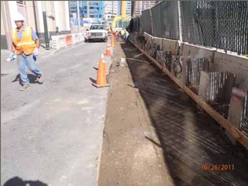
Preparing for Asphalt Replacement
