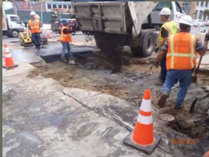
First Street Repairs
