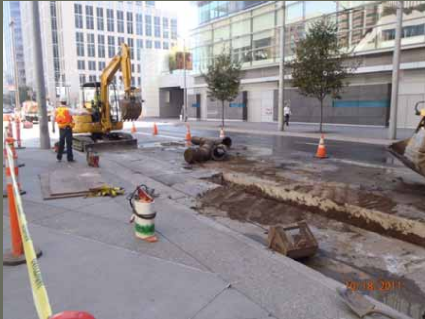
Pavement Restoration on Beale Street
