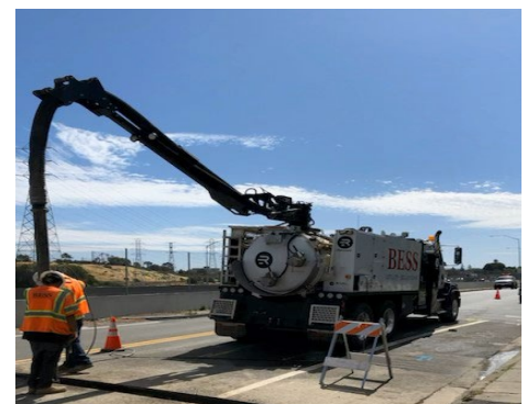
Figure 3. Vacuum truck used in excavating slot trench
