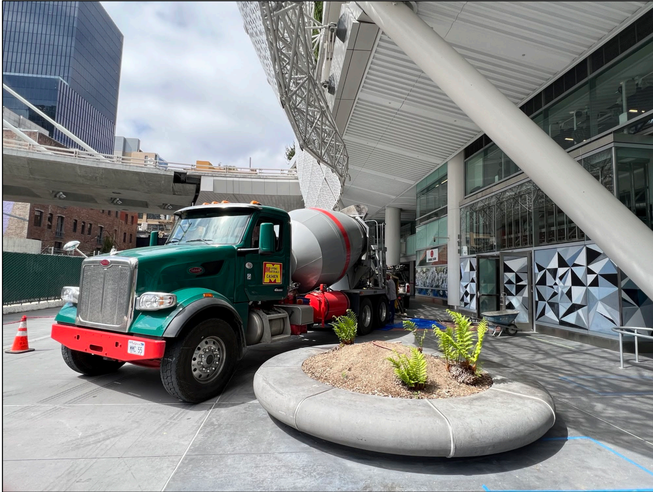
Via Vai; Concrete being poured
