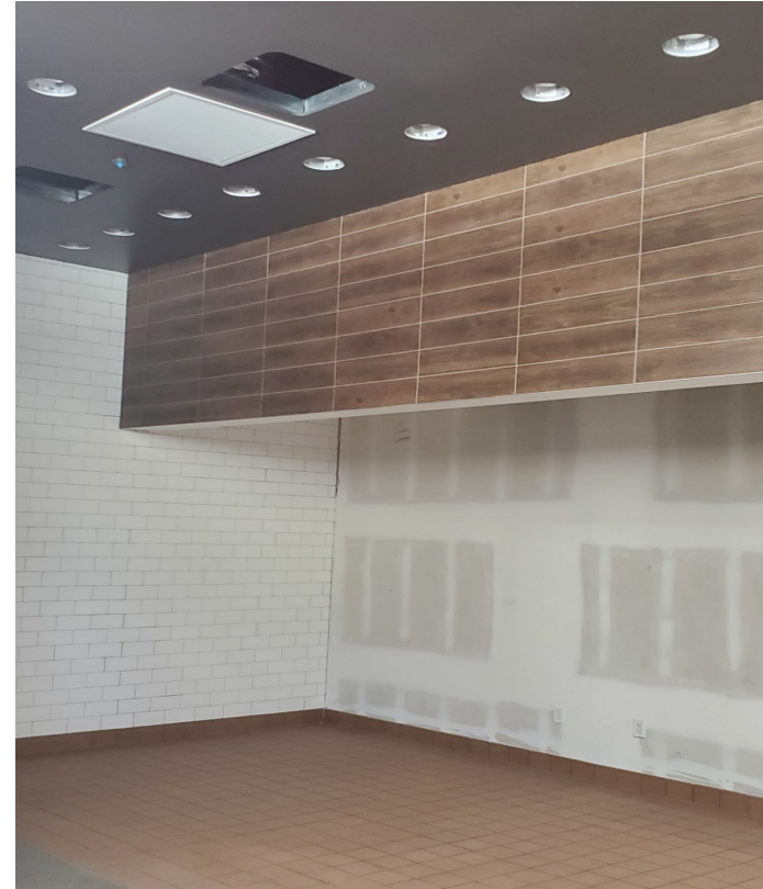
Charley's – ready for tenant buildout
