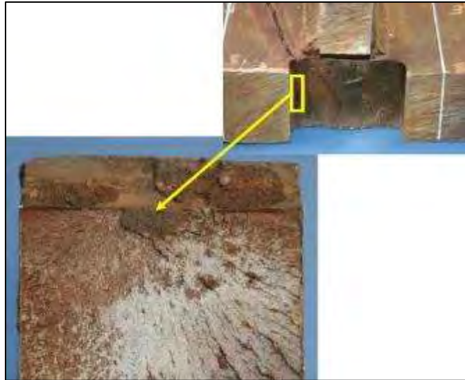
Fig. 12. Dark oxide covered elliptical pop-in crack fracture origin at the weld access hole (top) of girder sample D.4-NW.
