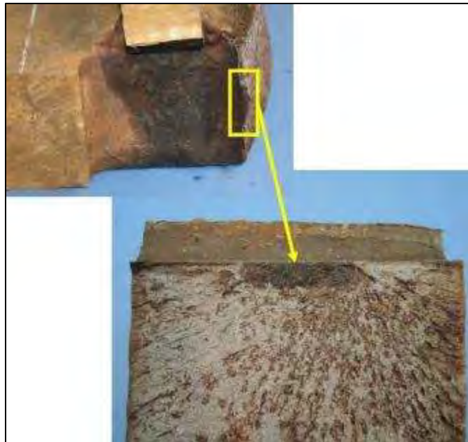
Fig. 13. Dark oxide covered elliptical pop-in crack fracture origin at the weld access hole (top) of girder sample E.6-SW.
