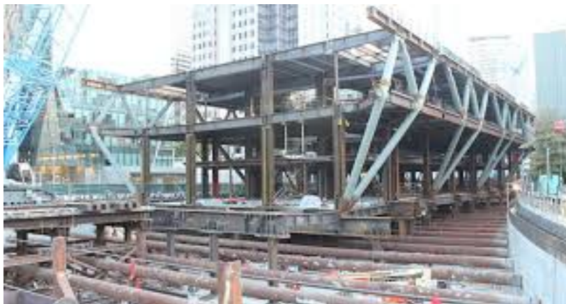
FIGURE 1 Construction of Transbay Transit Center
