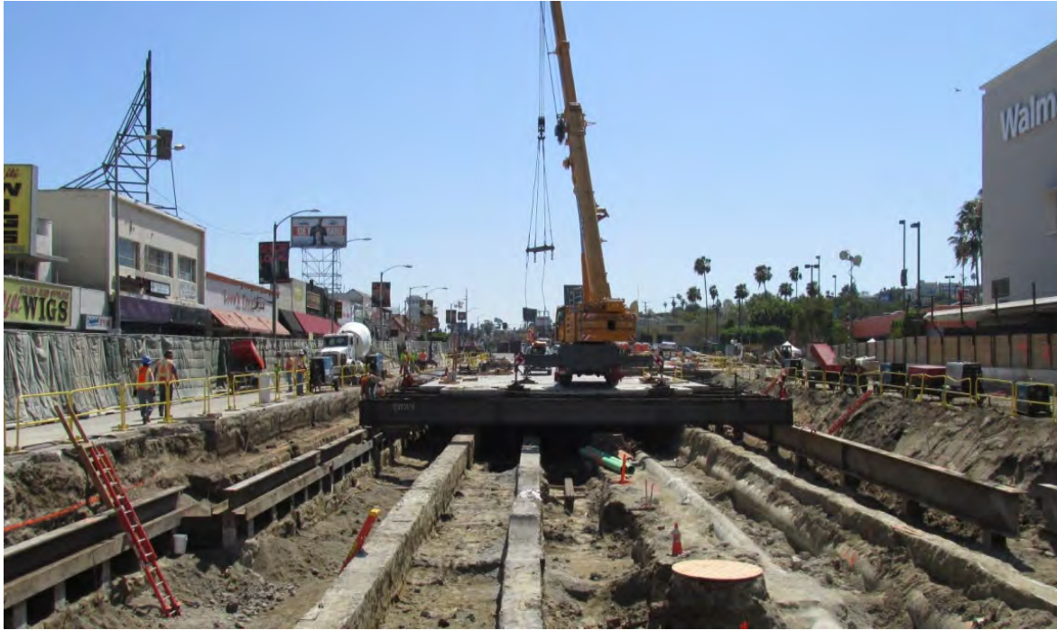
Figure MR-2. Photograph of Decking Installation
