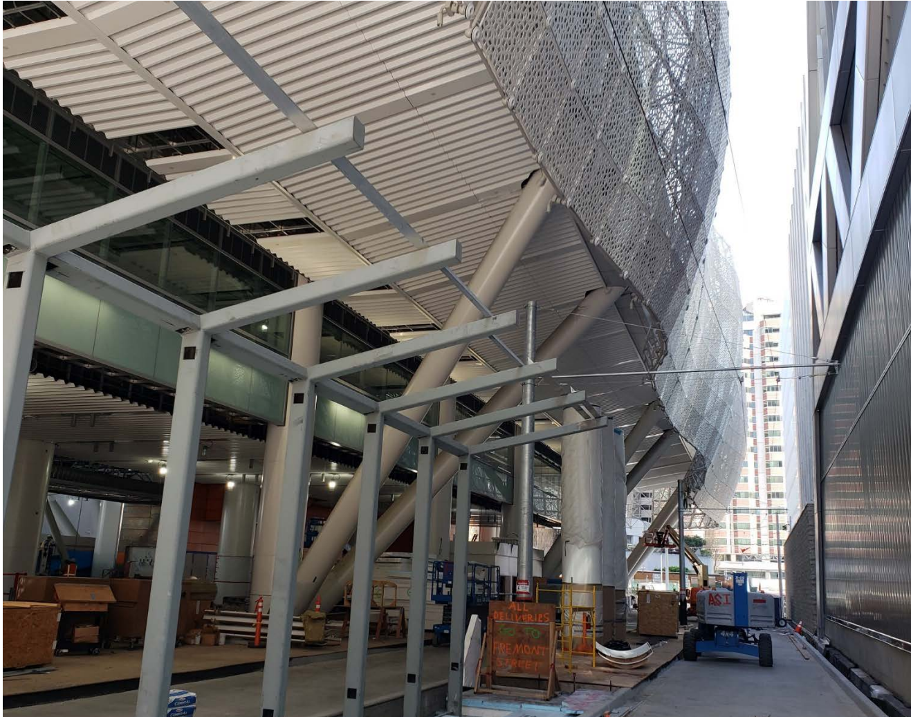
Muni Bus Plaza – south side progress
