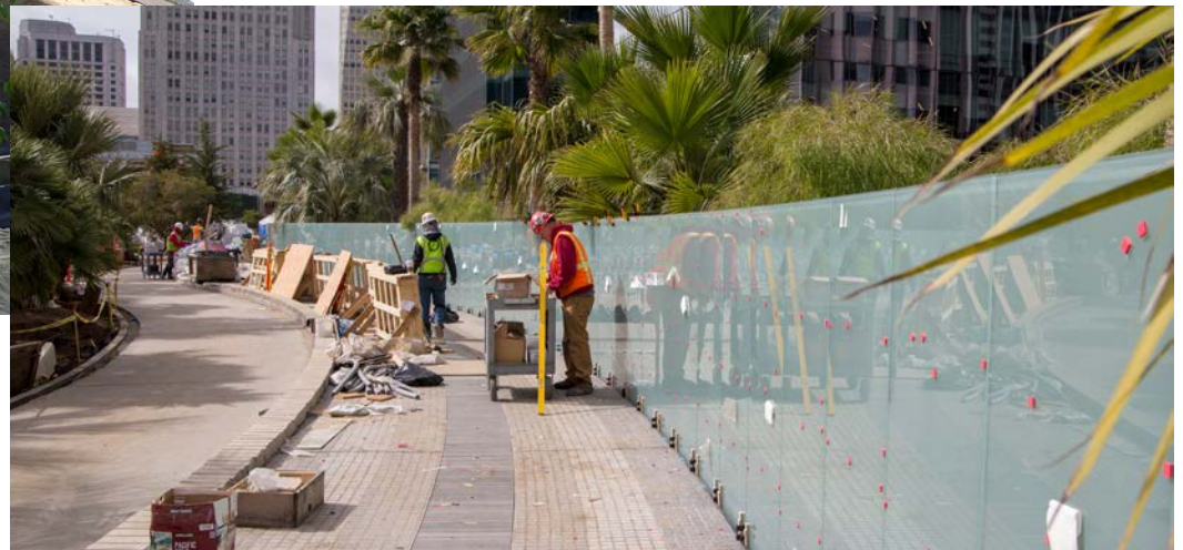
Bus Jet Fountain progress
