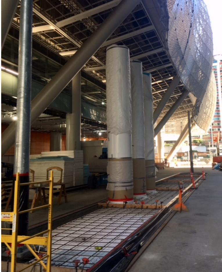
Muni Bus Plaza – South side progress
