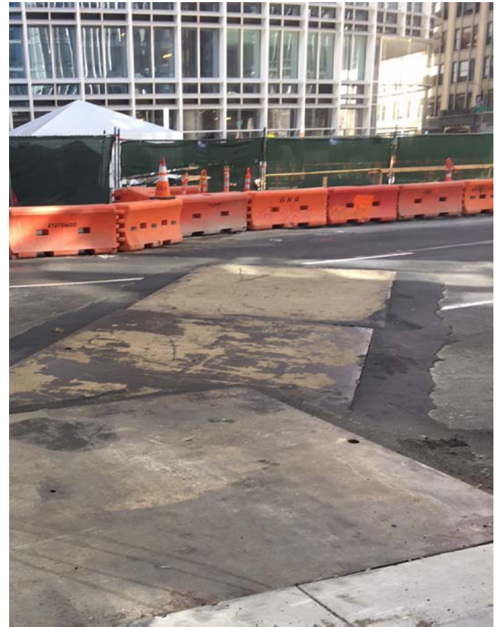
Muni Bus Plaza and Fremont Street storm drain connections
