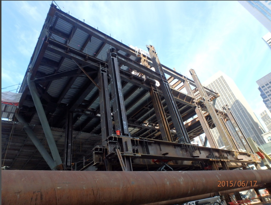
Above : Steel erection begins in the eastern zone.
