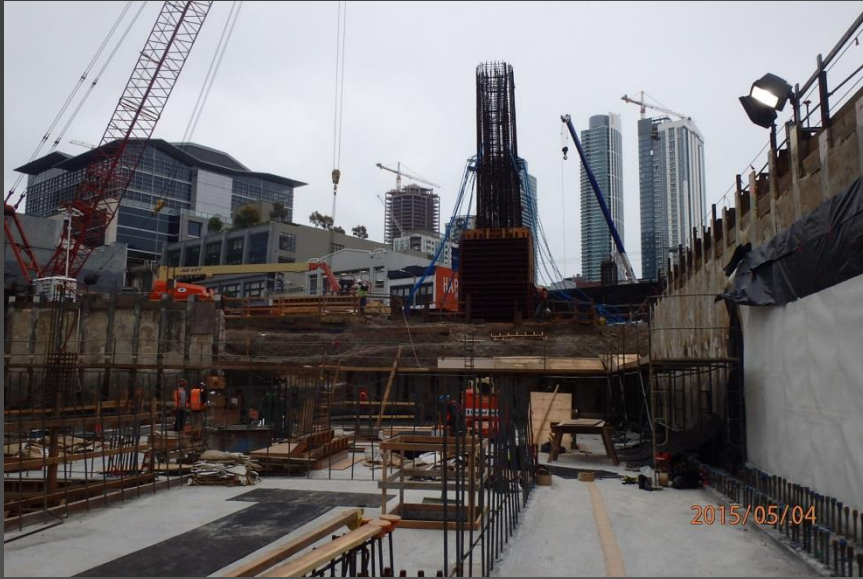
Above : Looking south at Pylon 9 for Cable Stay Bridge.
