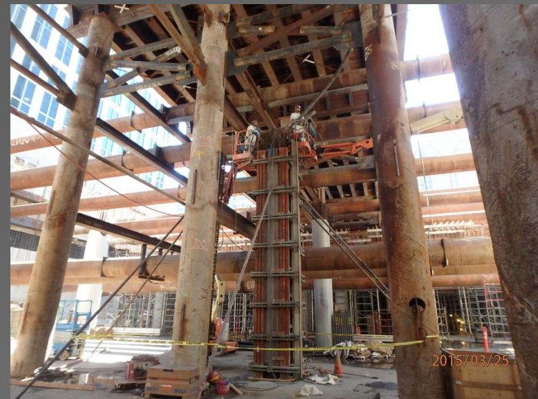
Above Right : RA level bracing at 3 rd lift walls.
