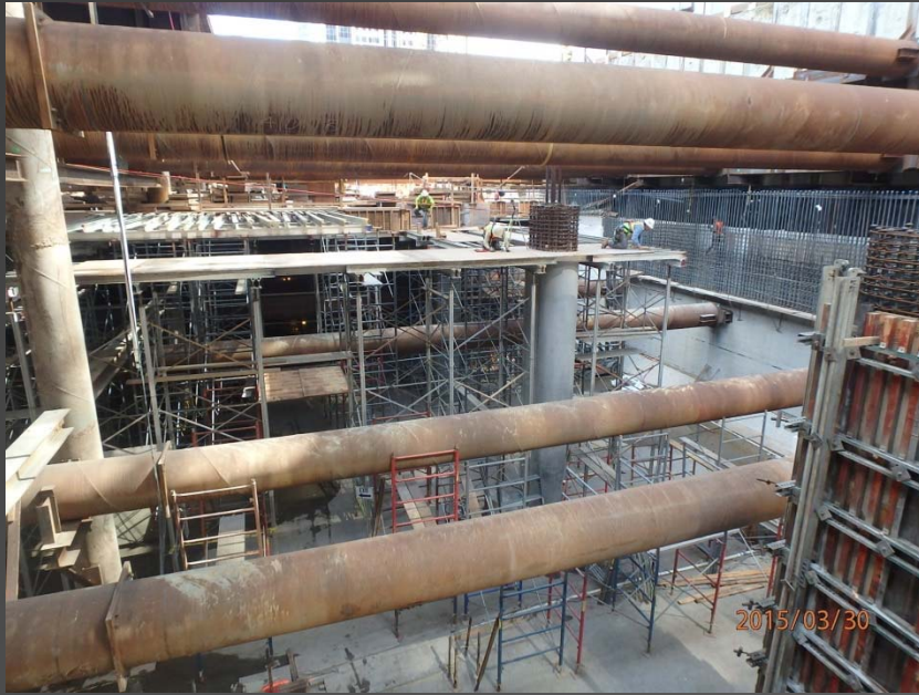
Above : Formwork for ongoing Lower Concourse work.
