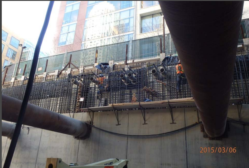
Above Left : Work progressing on fourth lift walls including future utility penetrations.
