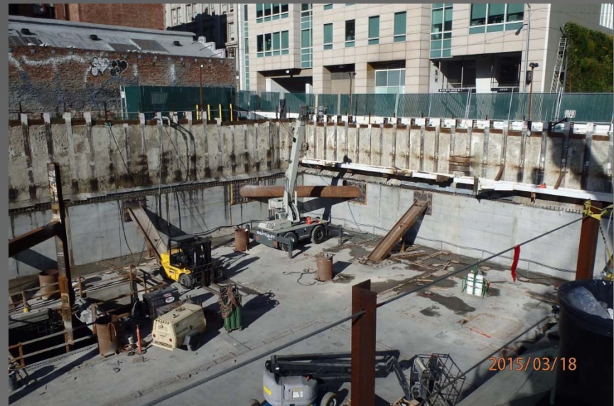
Above Left : Work progressing on fourth lift walls including future utility penetrations.
