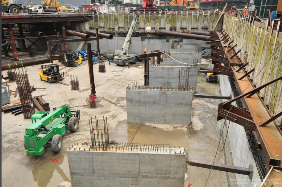
Above Left : Bracing removal at southwest corner of the project.
