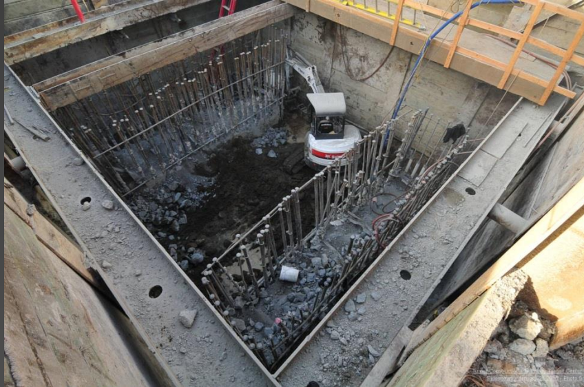
Above : Preparation of Pylon 9 for footing formwork.
