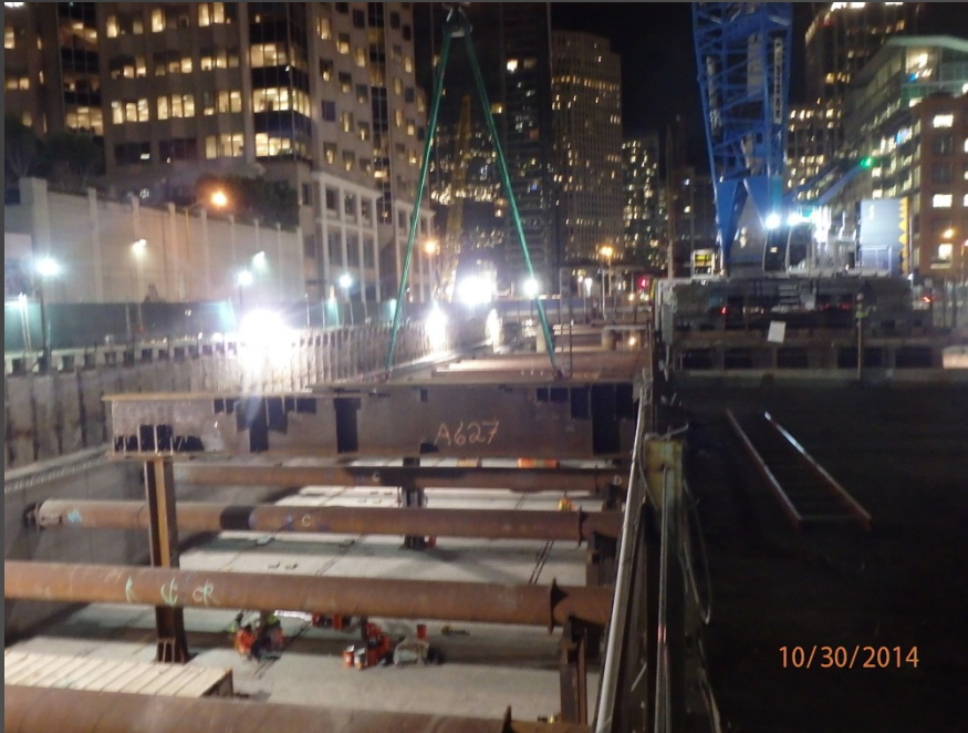
Left : Transfer Girder hoisted into place.
