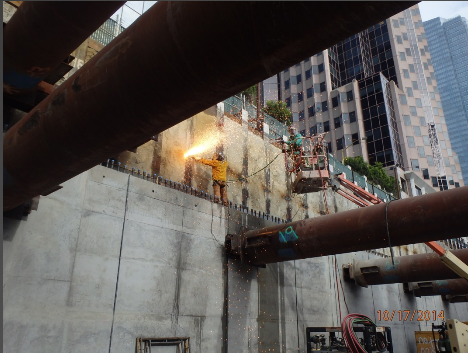
Above : Removing all Bracing Level A supports.
