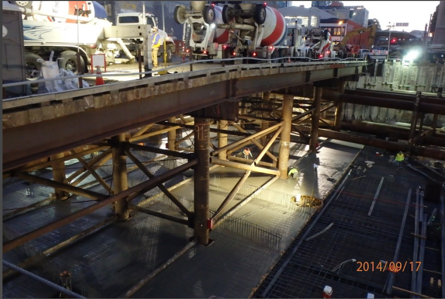
Left : Early morning Lower Concourse concrete pour.
