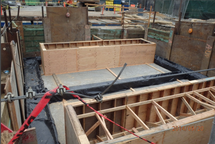
Left : Preparation for Pylon 9 Barrette Pile.
