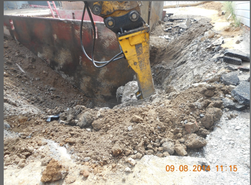
Right : Demolition and preparation for CIDH piles.
