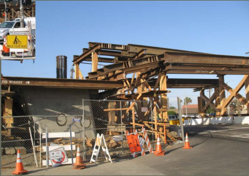
Typical roadway falsework
