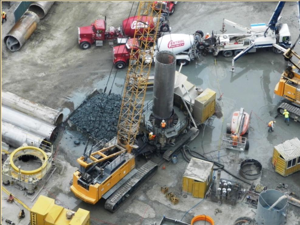
CIDH starter casing installation
