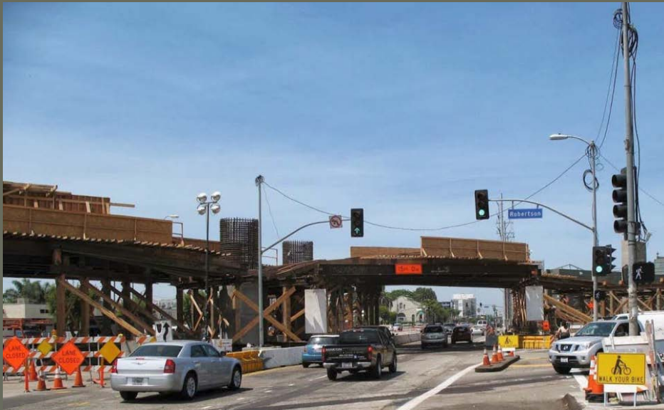
Typical roadway falsework
