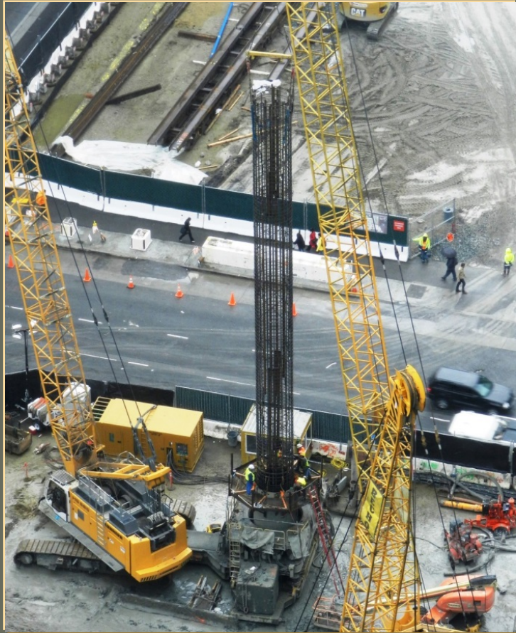
CIDH rebar cage installation
