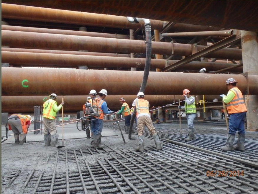
Mat Slab #12 Placement.
