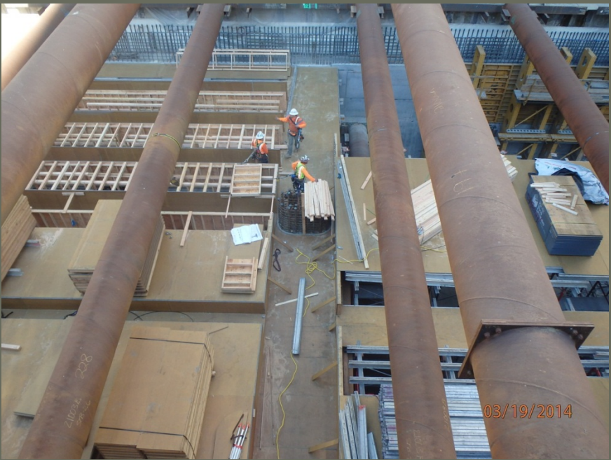
Lower Concourse Slab Forming Continues
