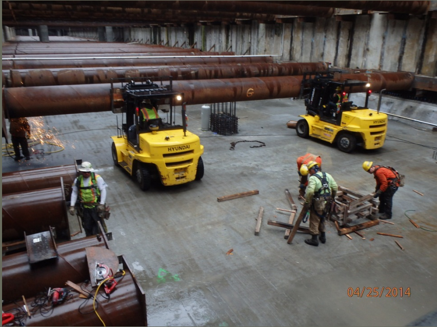
Second Foundation Wall Lift and Re-Bracing Continues
