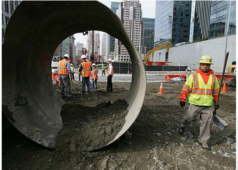
Transbay Terminal Construction
