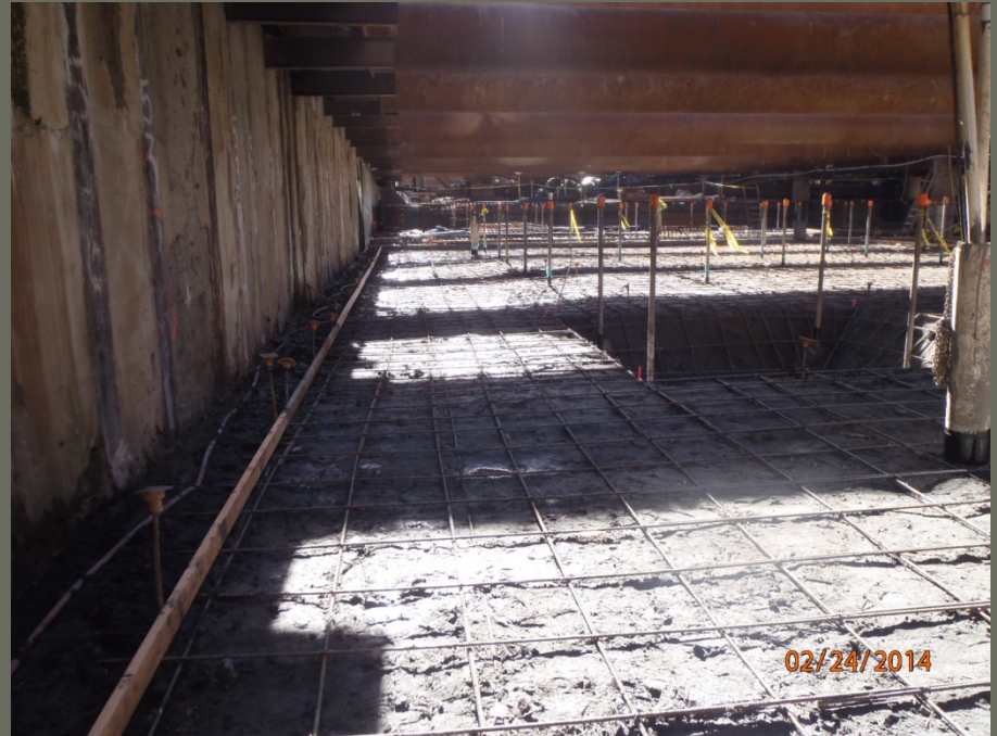
Sub grade and mud slab preparation
