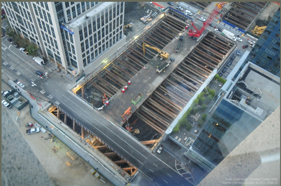
Turner Construction Co. Transbay Transit Center Edgar J. Overview, October 30, 2013 - Photo 19
