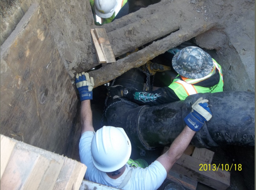
First Street intersection completed
