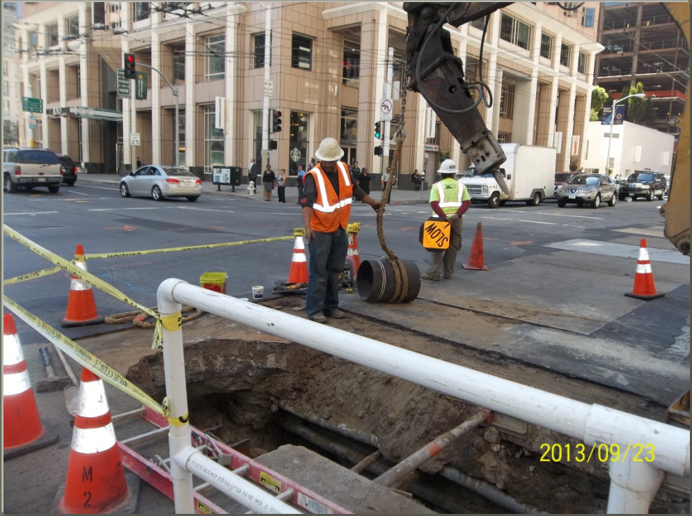
Work at First Street Intersection
