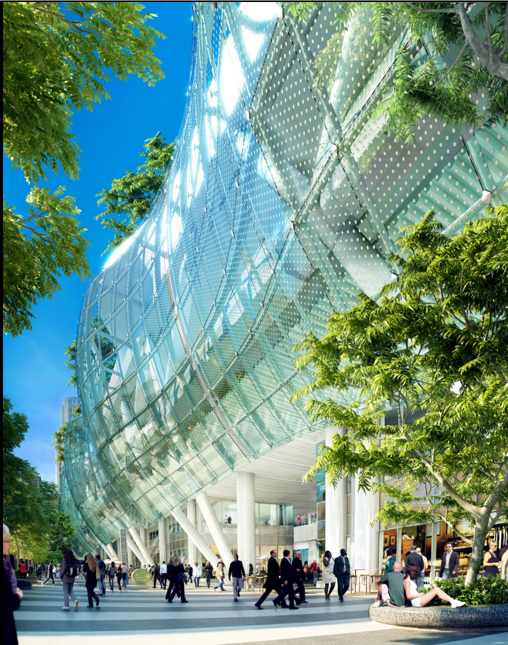
NATOMA STREET VIEW – GLASS AWNING
