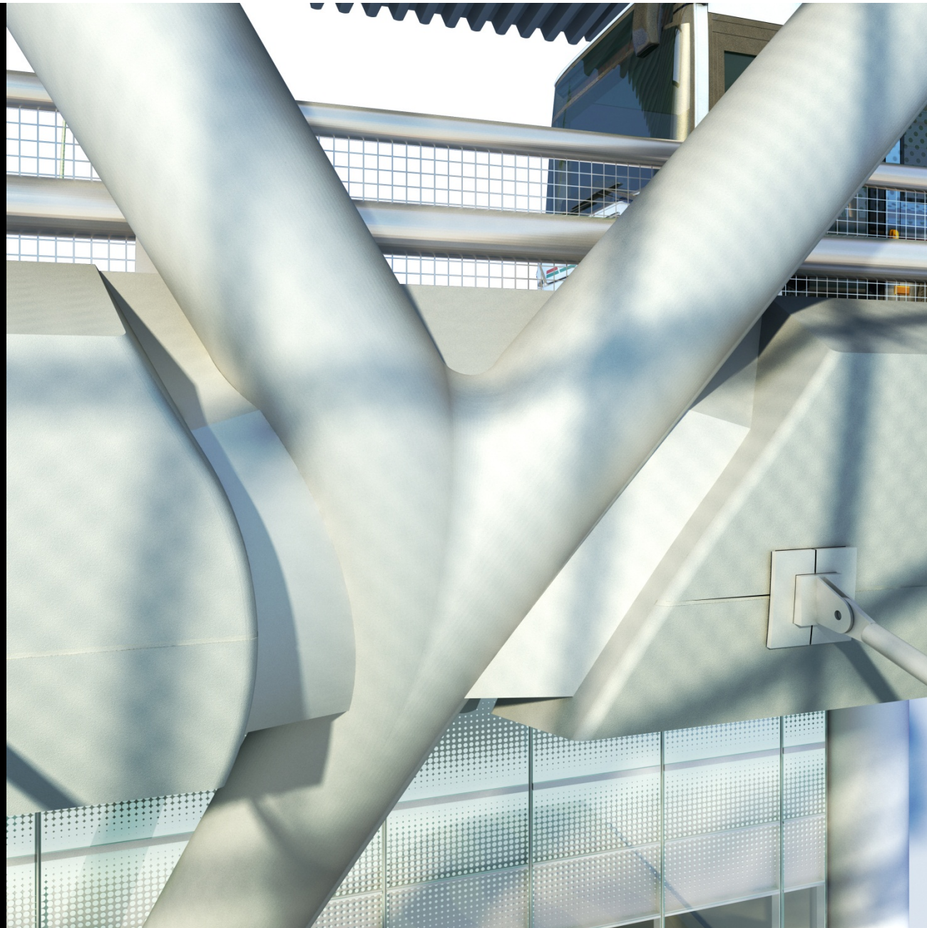
SUPERSTRUCTURE CONNECTIONS AT BUS DECK
