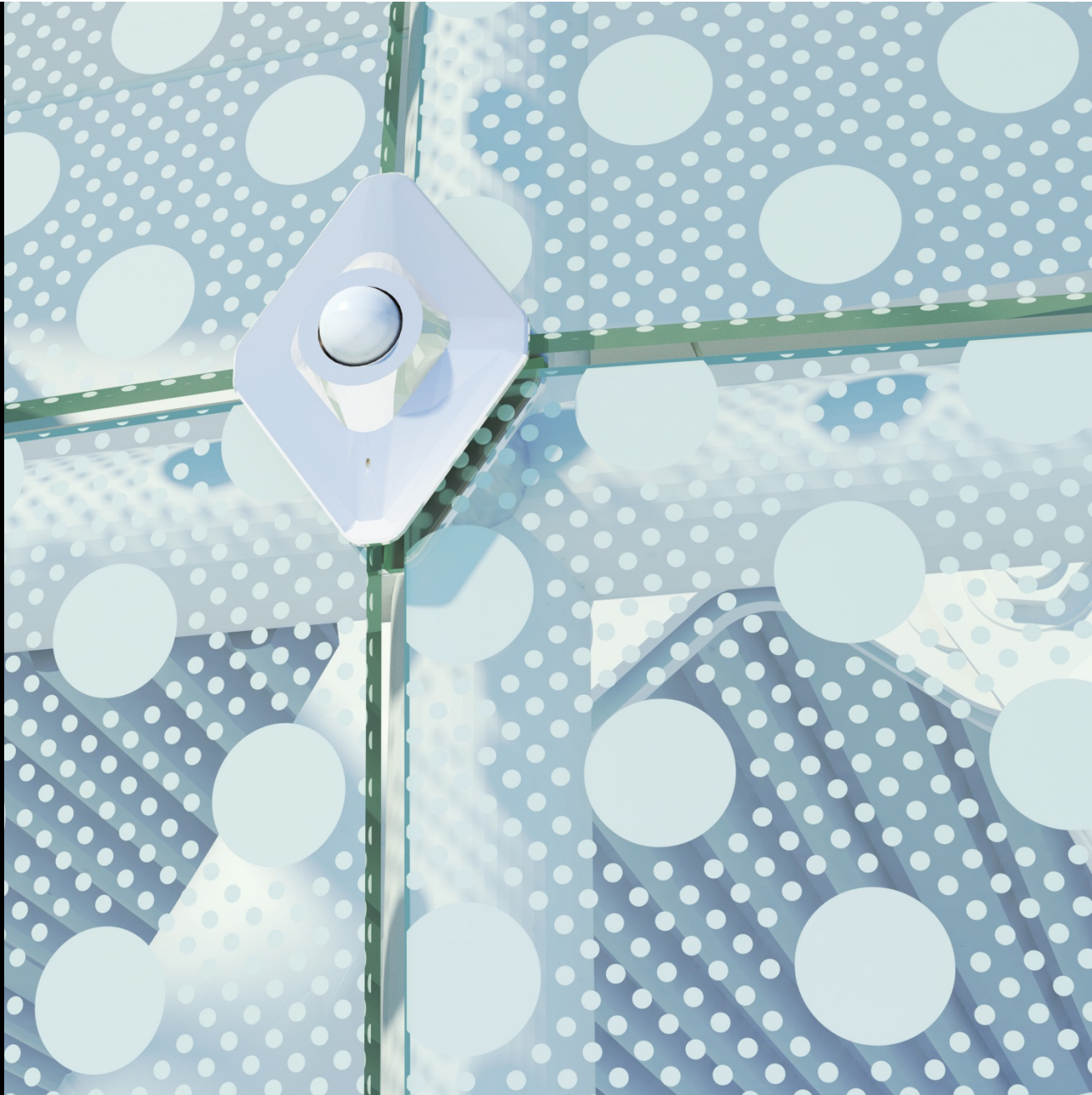
GLASS AWNING DETAIL AT PATCH NODE
