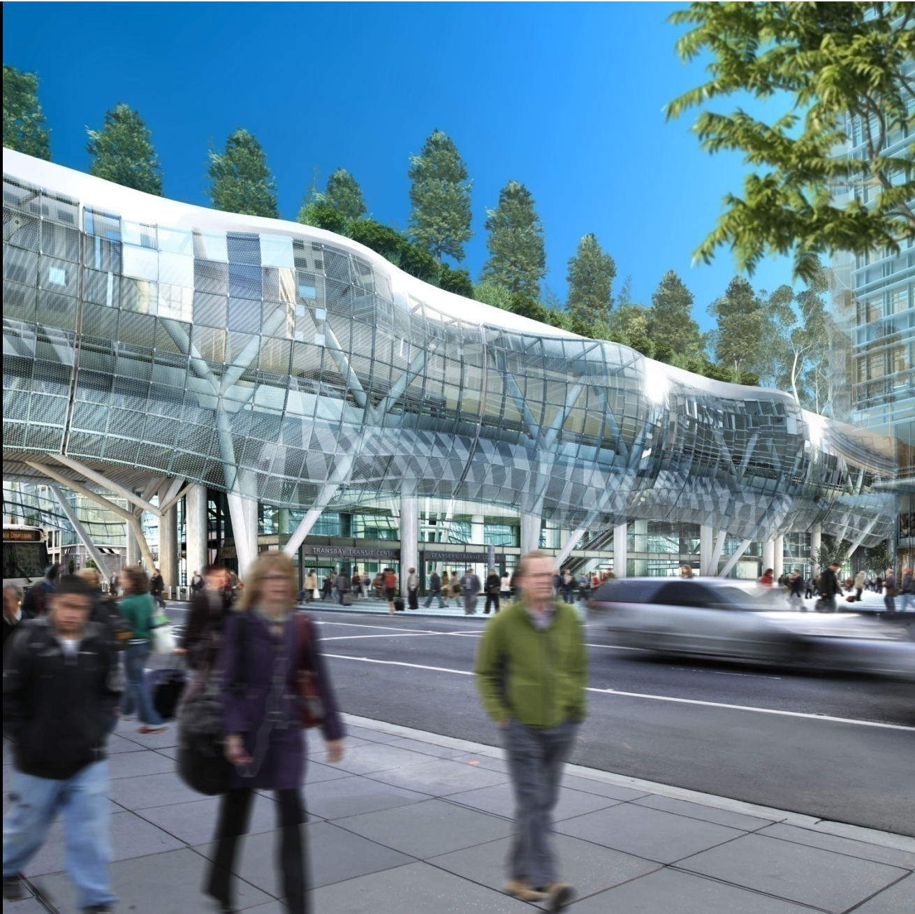
FREMONT STREET & MISSION SQUARE VIEW
