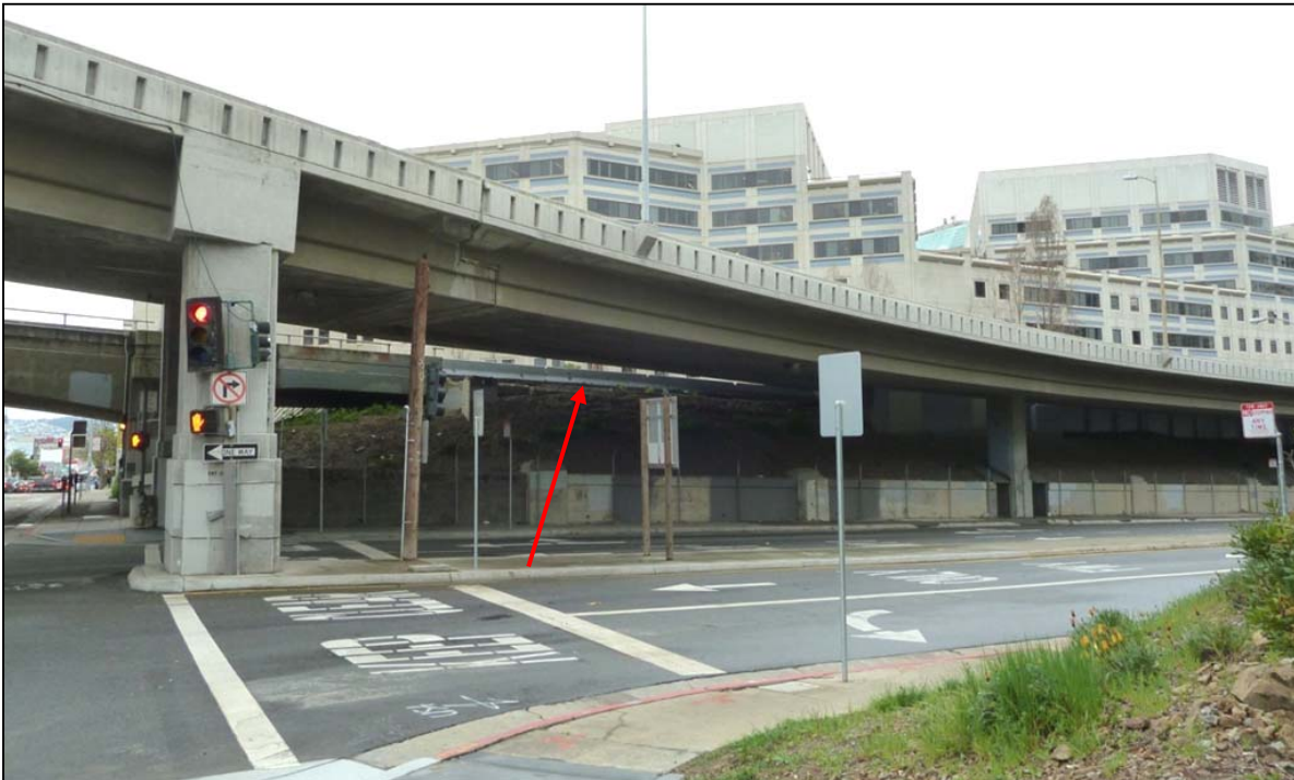
Photograph 2: Portion of the former Transbay Terminal Bus Ramp that passed through the Project Area prior to its demolition. Fremont Street exit ramp in foreground remains and is not historic. Camera facing southwest, JRP April 2011.
