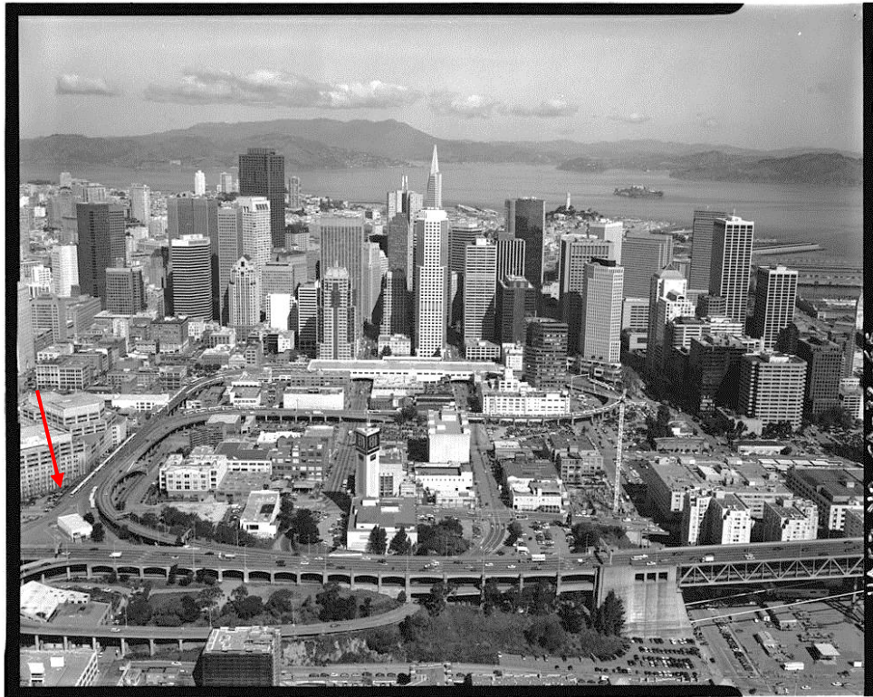
Photograph 1: Overview of Transbay Terminal Bus Ramp, 1985 San Francisco-Oakland Bay Bridge HAER
