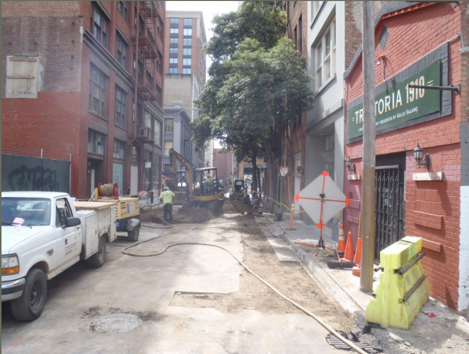
Pavement Restoration, Natoma at 2 nd Street
