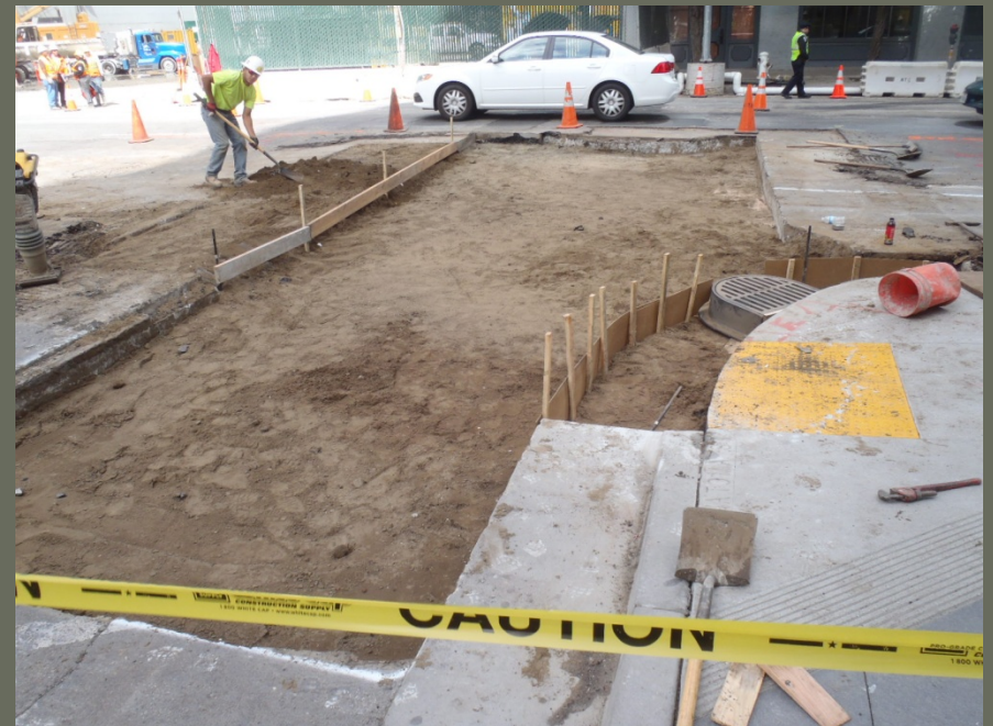
Pavement Restoration, Natoma and Fremont
