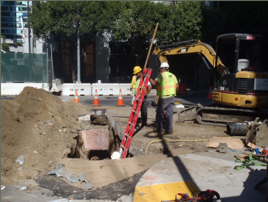
Sewer install, Natoma and Fremont
