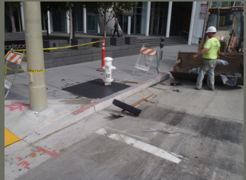
Sidewalk Restoration, Howard Street
