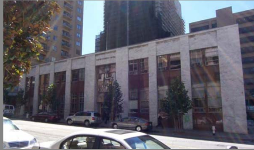
Marine Fireman's Union Building (240 2 nd Street, Built 1957)
