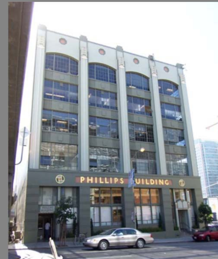
Phillips Building (234 1 st Street, Built 1929)
