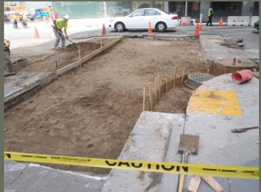
Pavement Restoration in progress, |Natoma and Fremont
