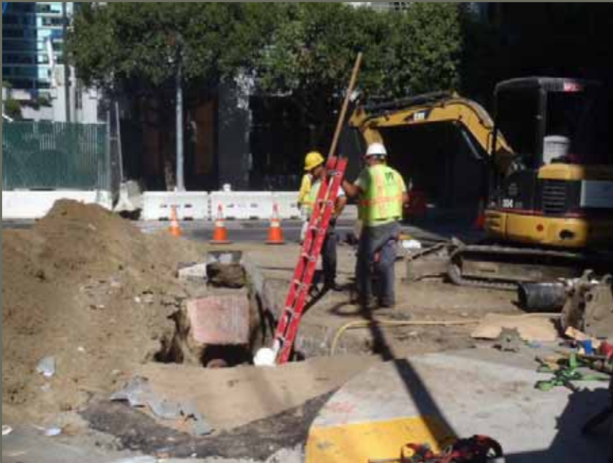
Sewer install, Natoma and Fremont
