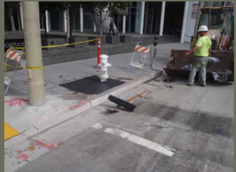
Sidewalk Restoration, Howard Street
