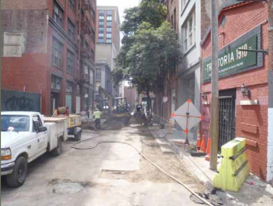
Pavement Restoration in progress, Natoma at 2 nd Street
