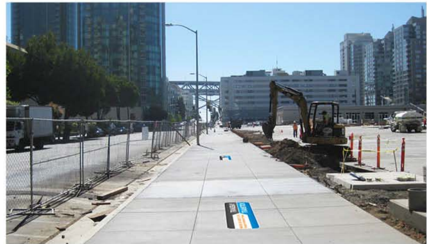
Transbay Temporary Terminal Main St Entrance
