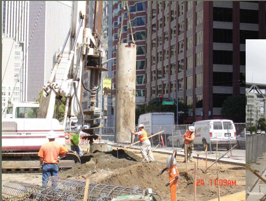
Canopy Foundations on Main St.
