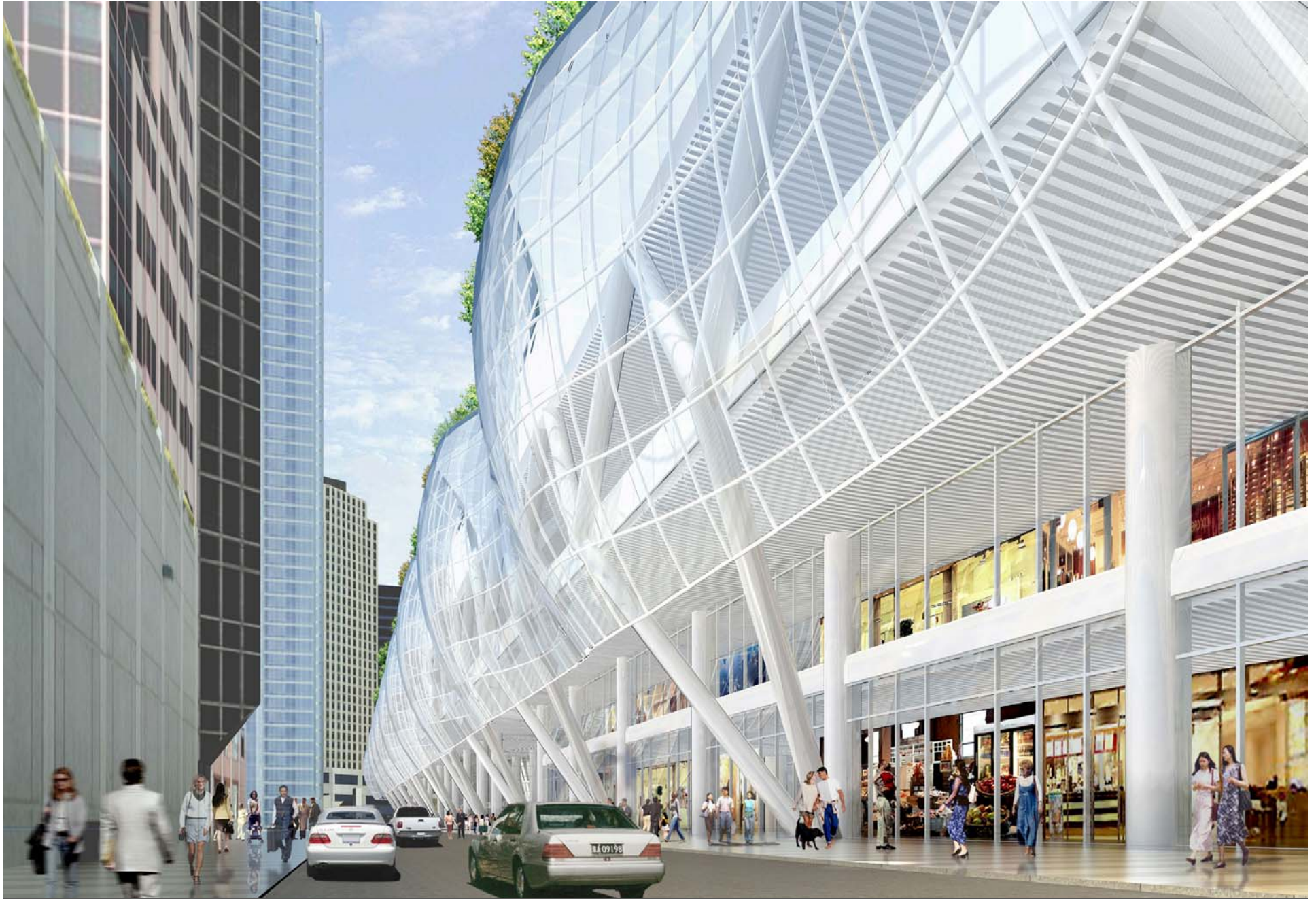
MINNA STREET VIEW LOOKING EAST
