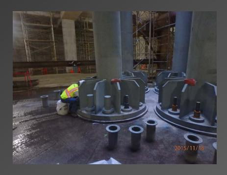
Above: Covering light column bolts after final testing.
