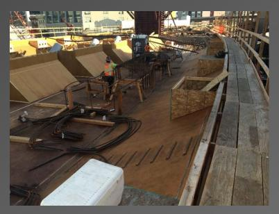
Above: Bridge formwork, looking south from the transit center at cable stay pylon 9.
