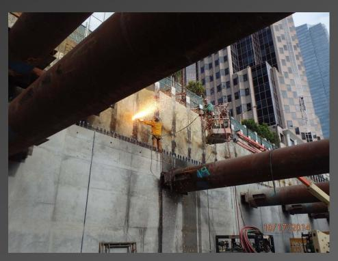
Above: Removing all Bracing Level A supports.
