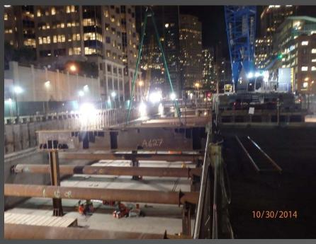
Left: Transfer Girder hoisted into place.
