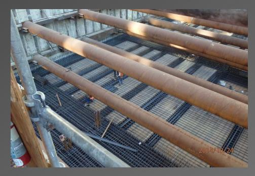
Above Left: Wall lift 2 reinforcing steel installation.
