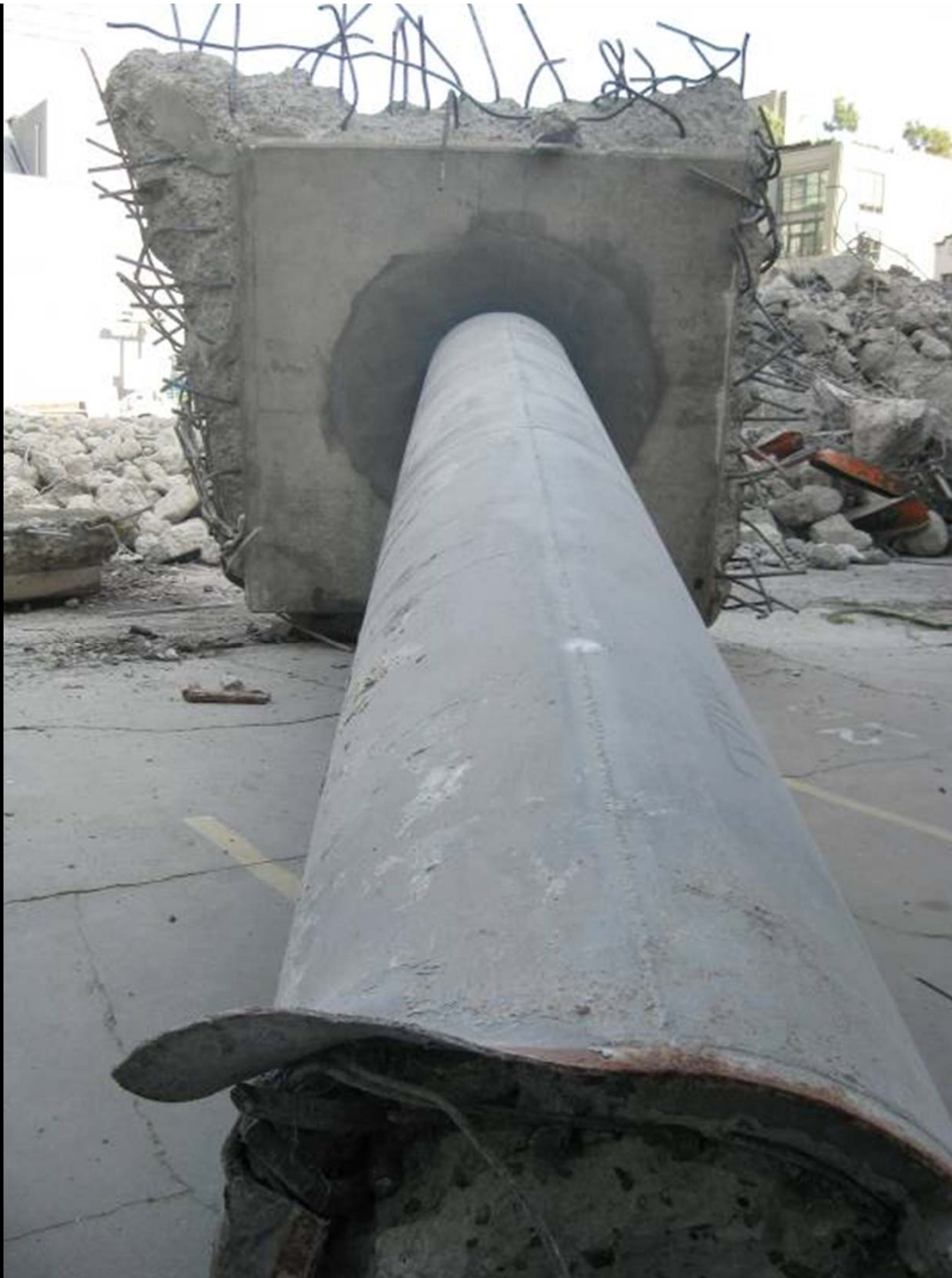
Left Arm from Phase III demolition
